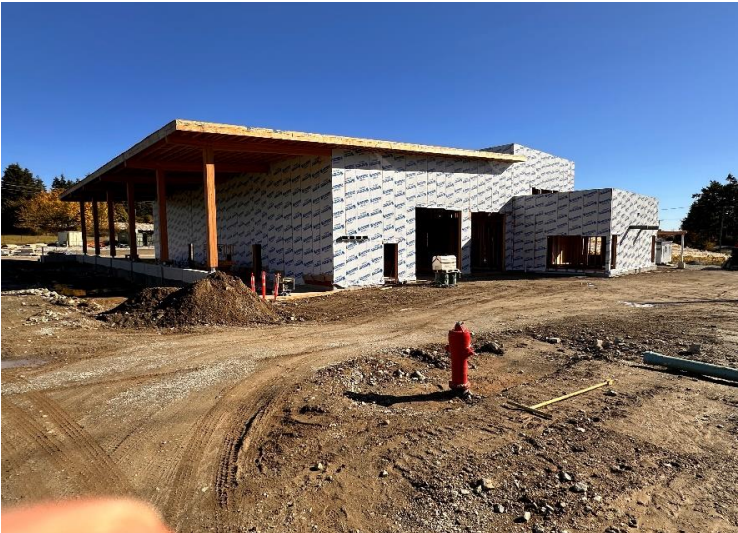
Vapour Barrier Installed
