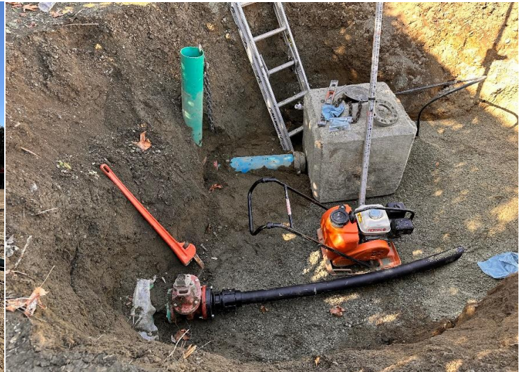
Water Connection Made to Main
