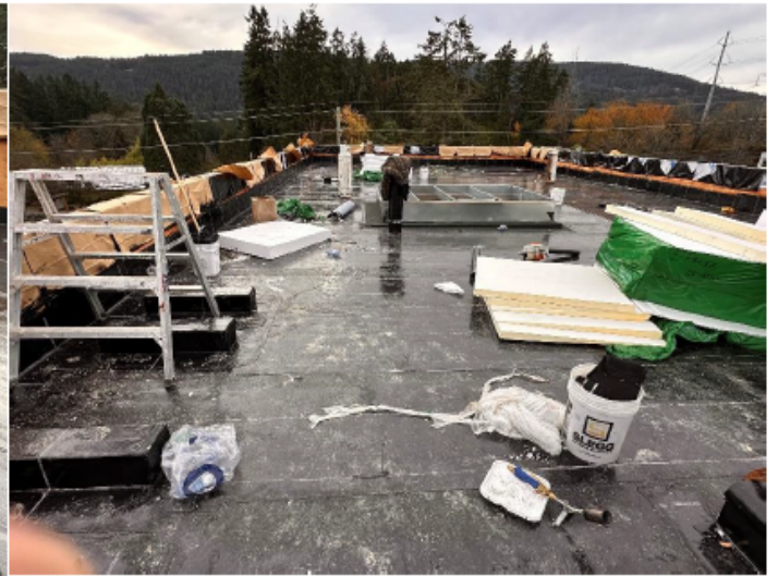
Upper Roof with Equipment Curbs
