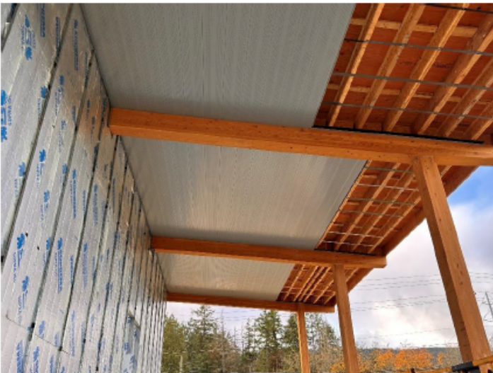
Soffits Being Installed
