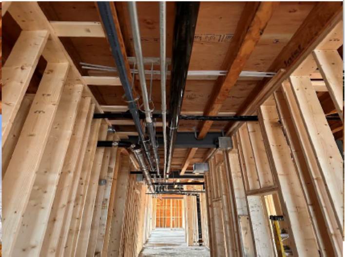
Plumbing and Mechanical Being Installed
