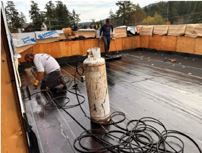
Roofing Being Installed on South Deck
