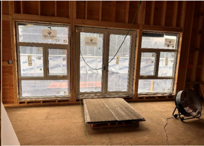
South on Second Floor
