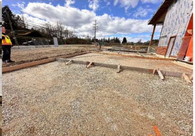
Front Apron Forms
