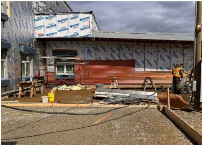
Cladding on South Wall
