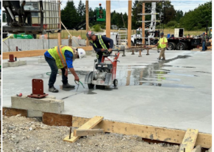
Cutting Control Joints
