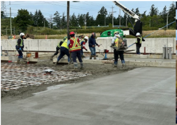
Slab Concrete Placing
