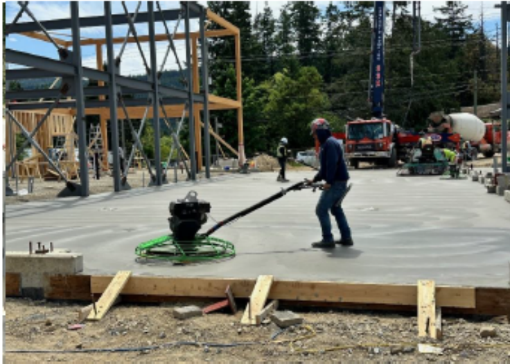
Concrete Slab Finishing
