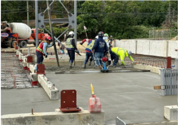
Slab Concrete Placing
