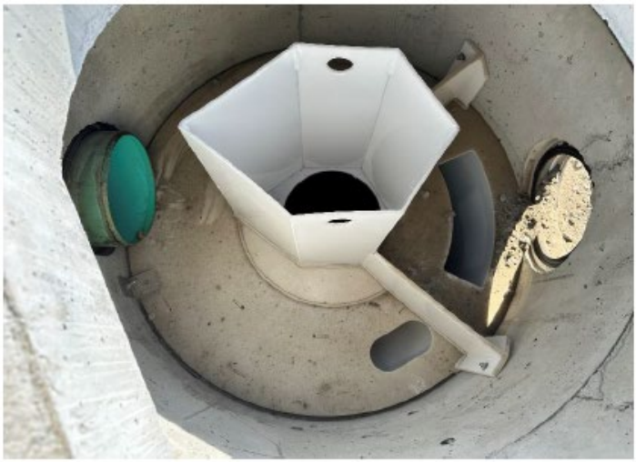
Oil Interceptor and Flow Control Management
