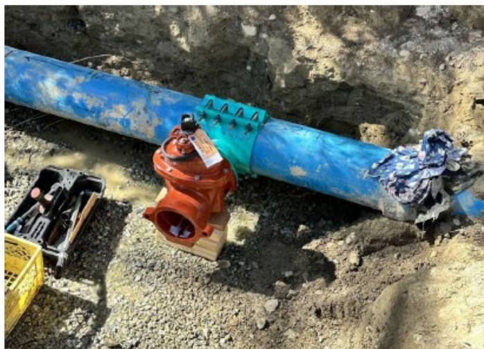
Completed 6" Valve Connection
