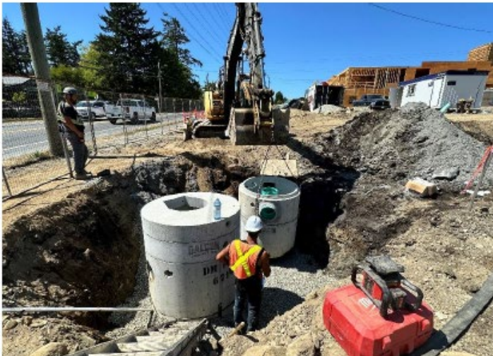
Installation of Stormwater System
