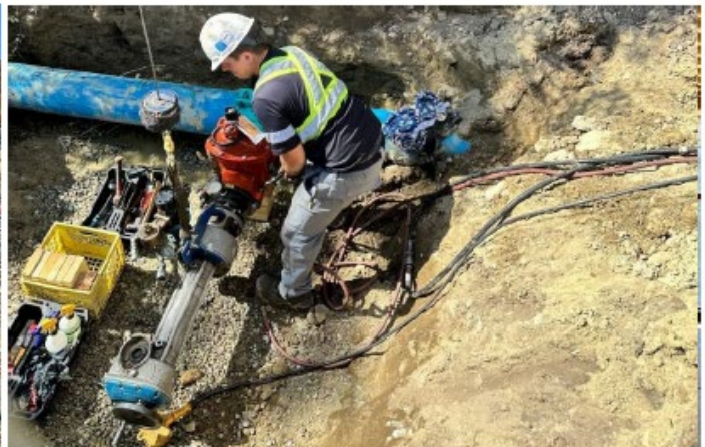
6" and 3" Hot Tabs Being Installed
