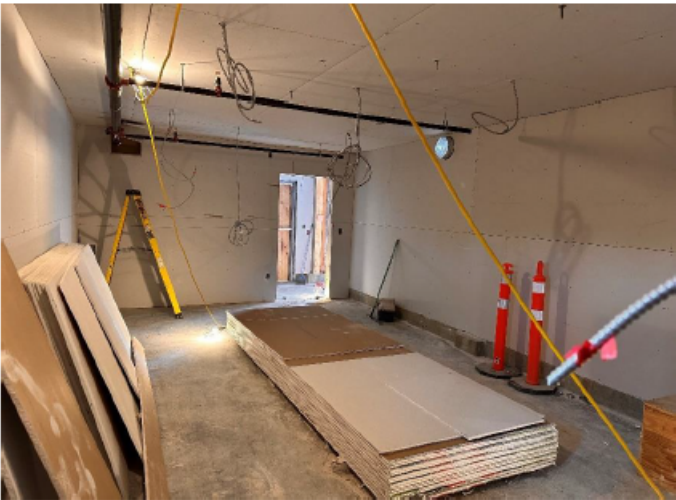
Lower Floor Drywall
