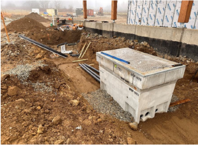
Hydro Under Ground work Installed
