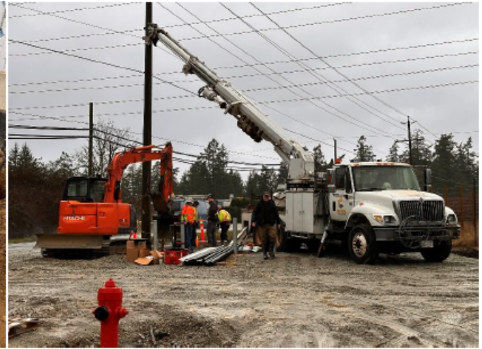
Hydro Install at the Pole
