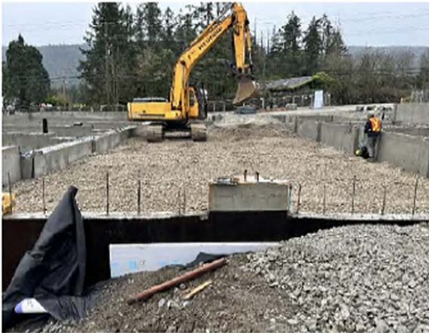
Infill of Foundation
