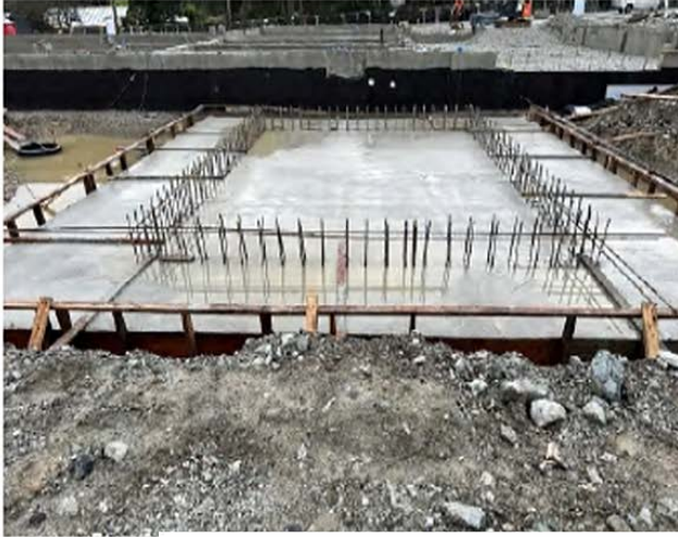
Hose Tower Raft Slab
