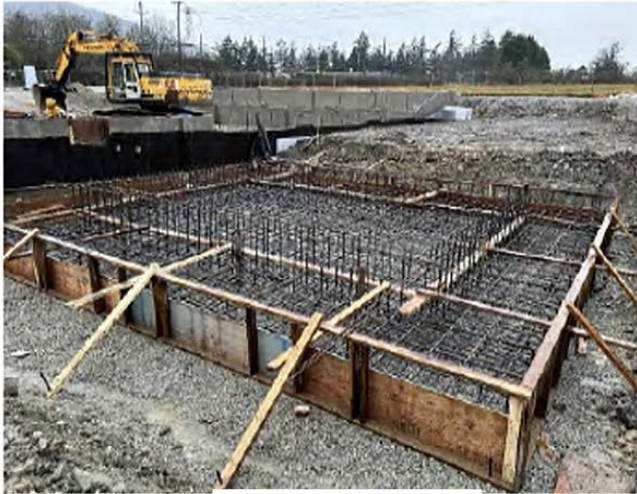
Hose Tower Raft Slab
