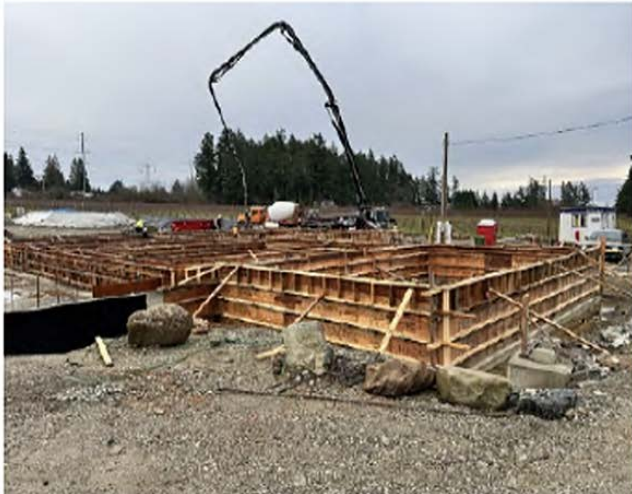
2nd Phase of Found. Wall Pour Dec 12th
