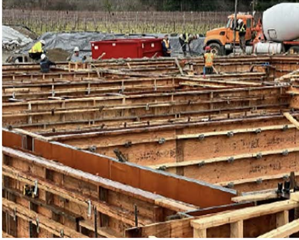
2nd Phase of Foundation Wall Pour Dec 12th
