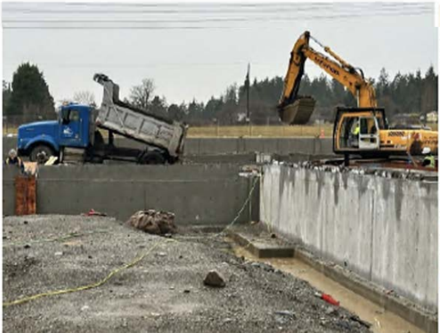
Infill of Foundation
