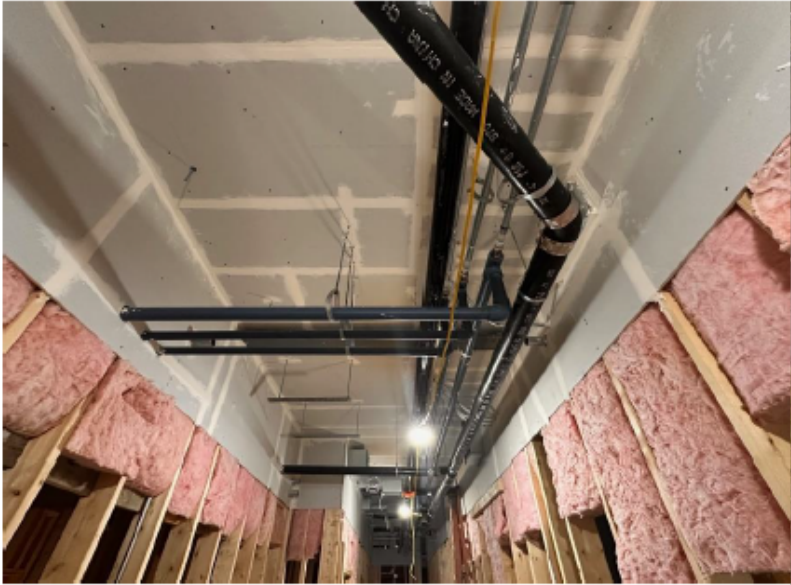
Insulation & Drywall in Corridor
