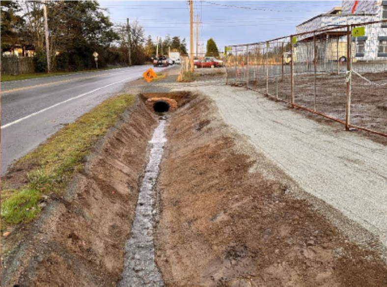
Restoring the Drainage Channel and Pathway
