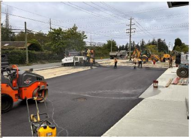
Front Apron Paving
