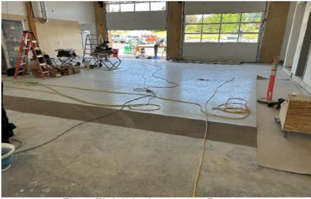
Floor Finish in Apparatus Bay
