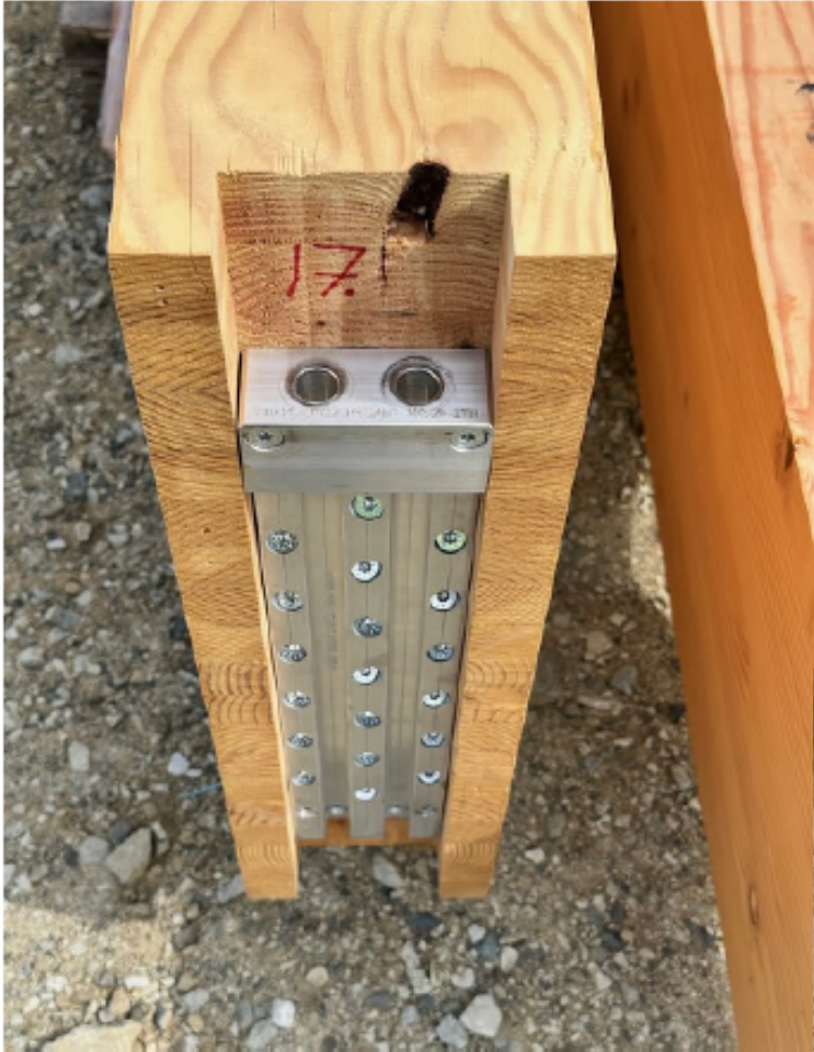
Timber to Timber Connection
