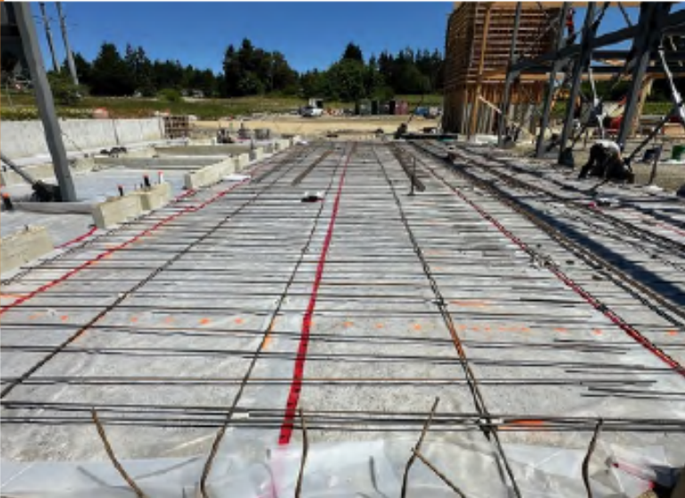
Installing of Reinforcing in Bay's
