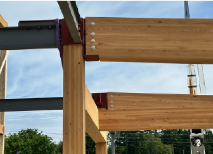
Timber to Steel Connection
