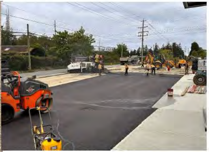
Front Apron Paving
