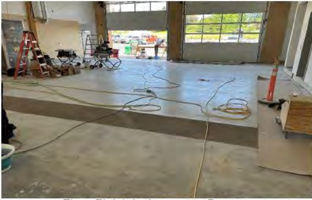
Floor Finish in Apparatus Bay
