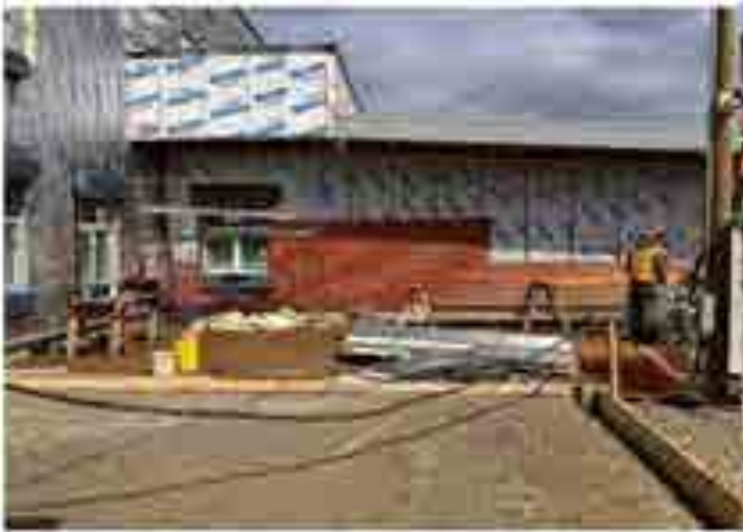
Cladding on South Wall
