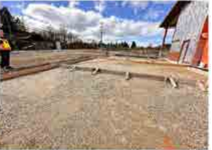
Front Apron Forms
