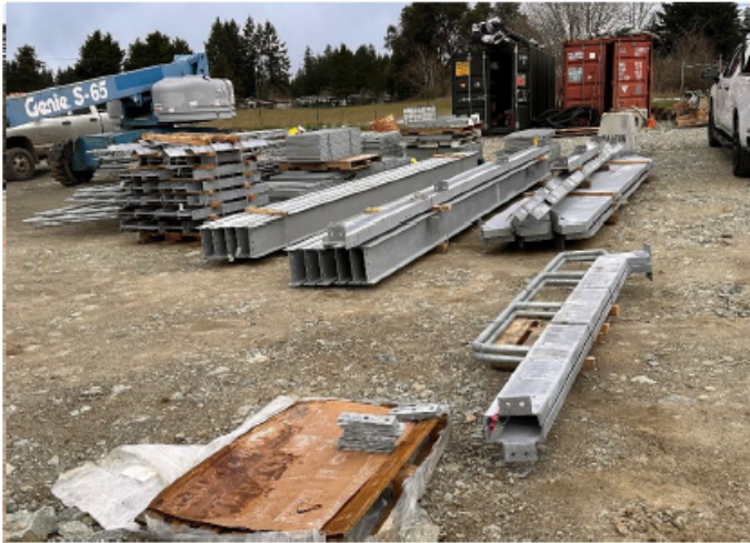
Galvanized Steel for Hose Tower
