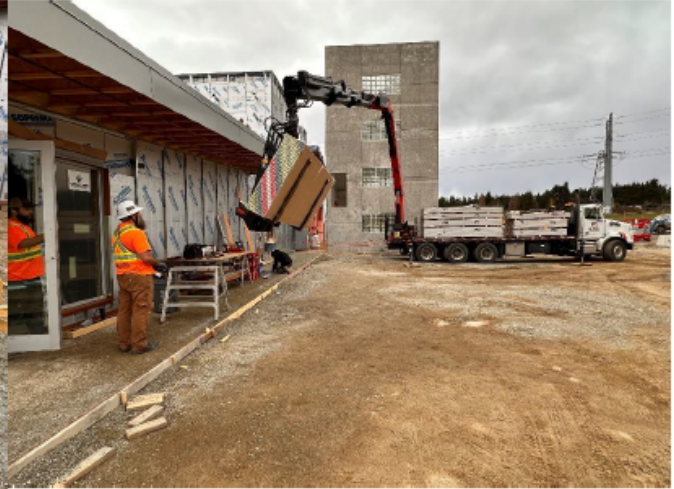
More Drywall Deliveries
