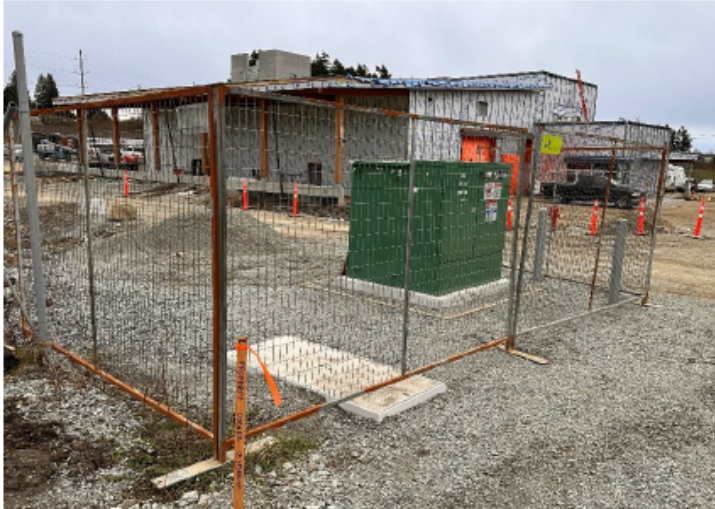
BC Hydro Transformer Installed
