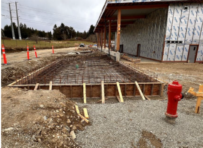
Cistern Tank Slab Preparation
