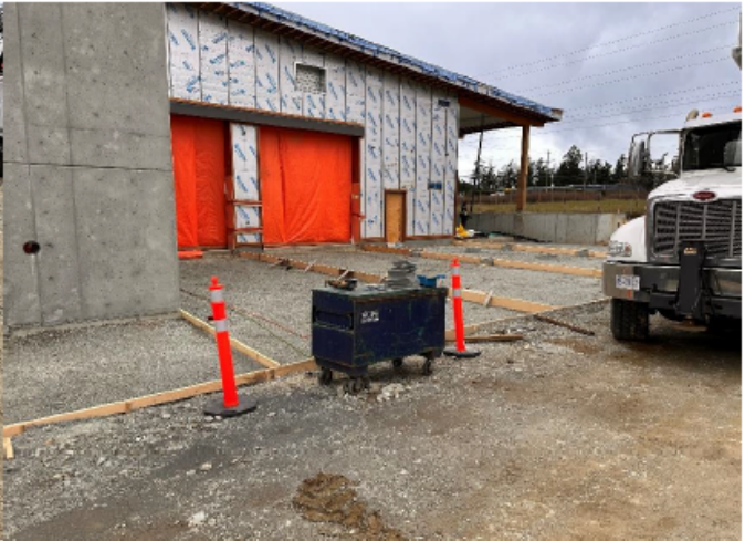
Rear Apron Slab Preparation
