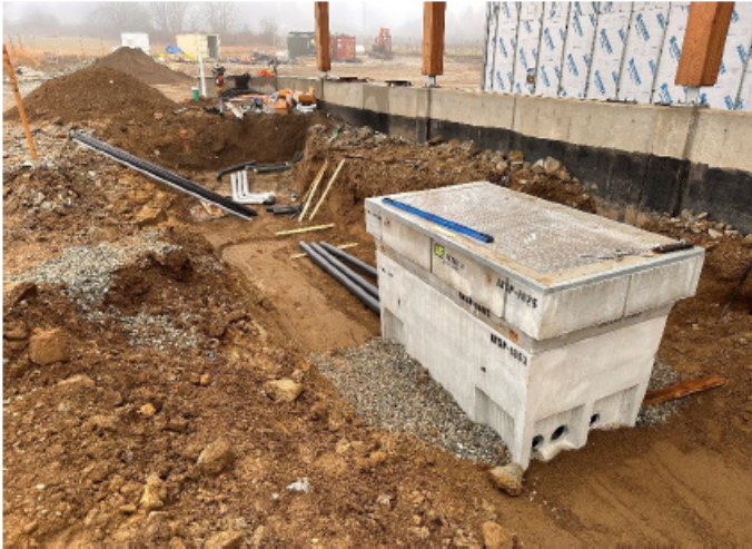
Hydro Under Ground work Installed
