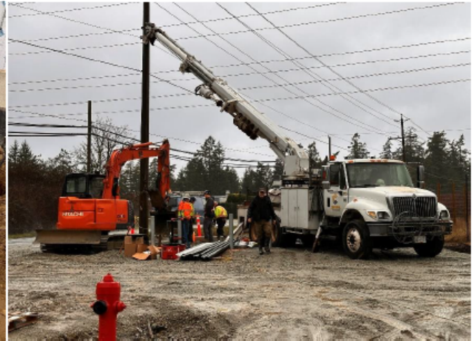
Hydro Install at the Pole
