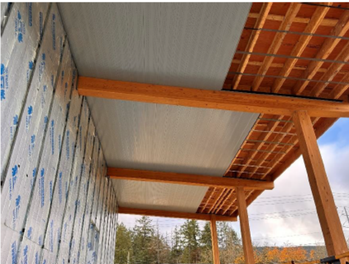
Soffits Being Installed
