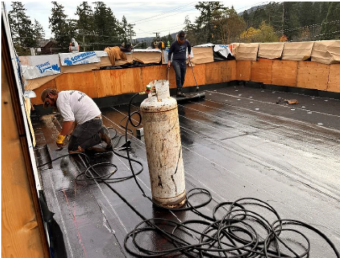
Roofing Being Installed on South Deck
