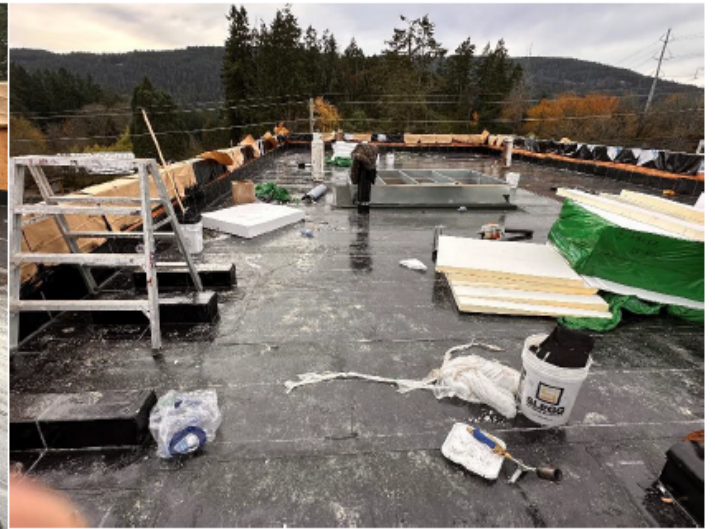
Upper Roof with Equipment Curbs
