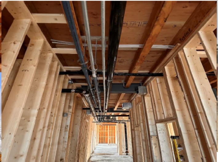
Plumbing and Mechanical Being Installed
