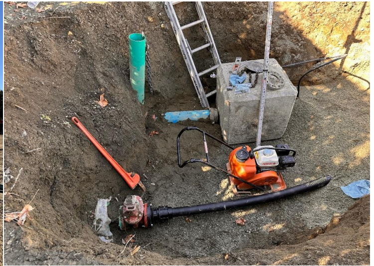
Water Connection Made to Main
