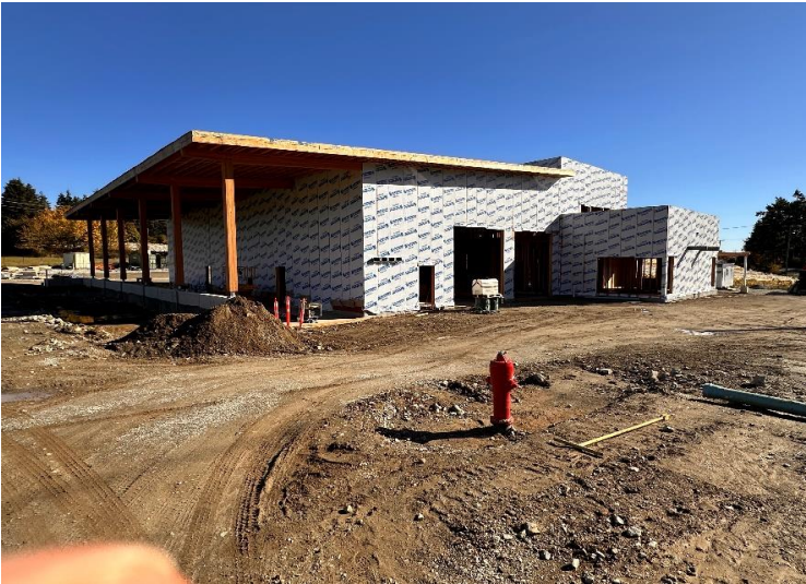
Vapour Barrier Installed
