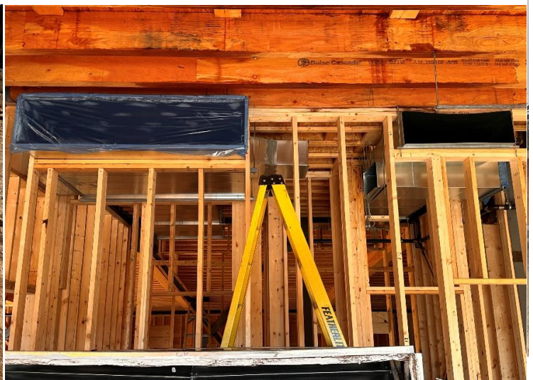
Plumbing and HVAC Duct Being Installed
