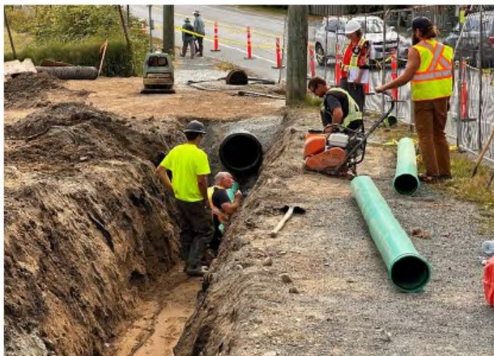
CRD Sewer Extension Connection
