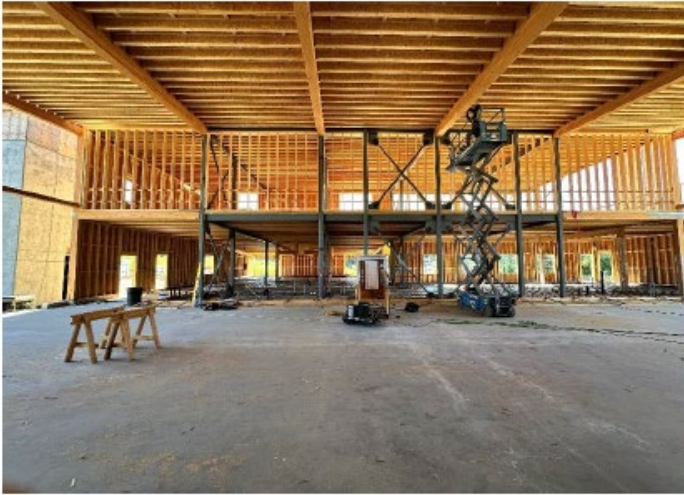
Roof Framing Over Bays
