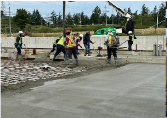
Slab Concrete Placing
