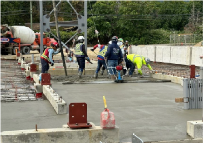
Slab Concrete Placing
