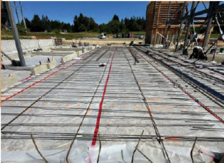
Installing of Reinforcing in Bay's
