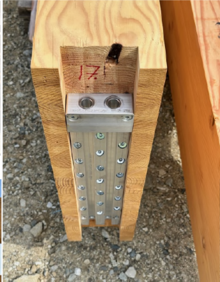
Timber to Timber Connection
