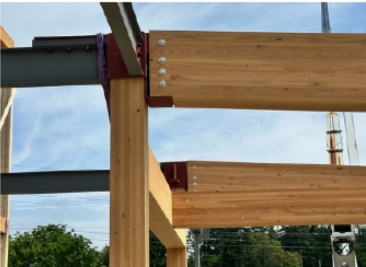
Timber to Steel Connection
