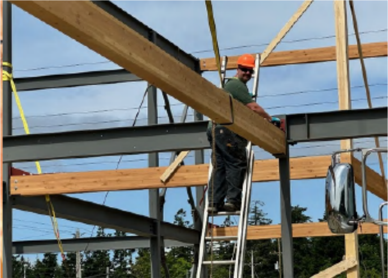
Placing of Another Beam
