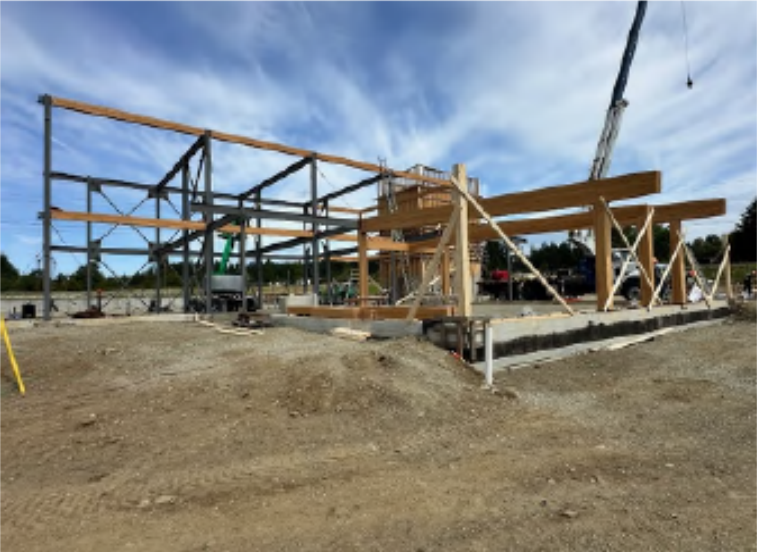
Portion of Timber Frame Completed
