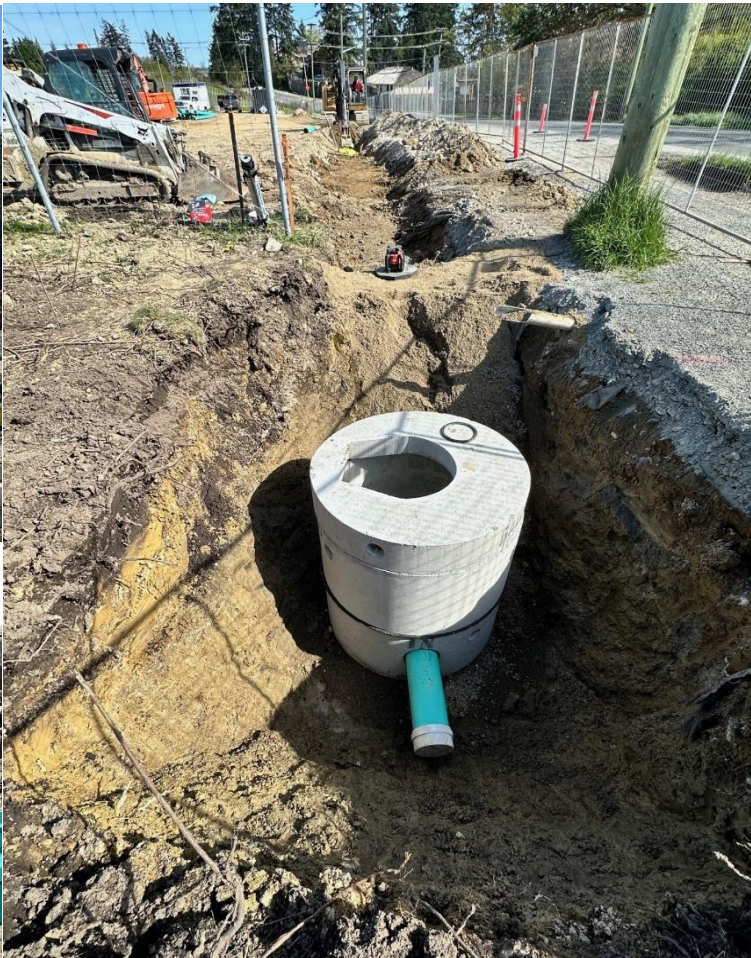
Sewer Line Install
